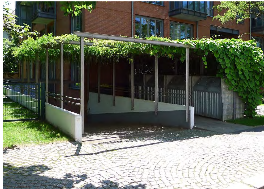
Screening to Basement Ramp
